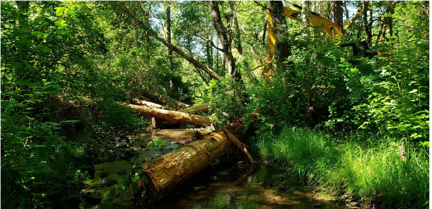
Large woody placement in side channels
