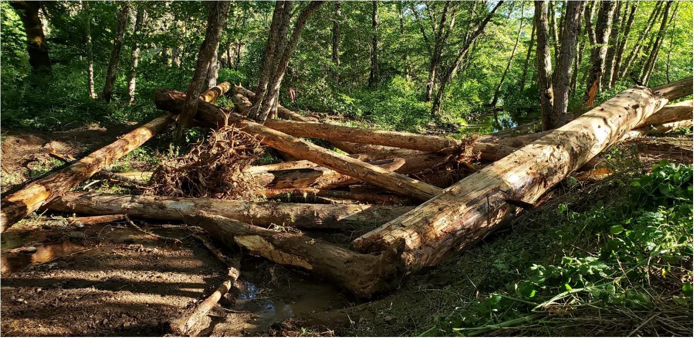
Large wood placement, finished product
