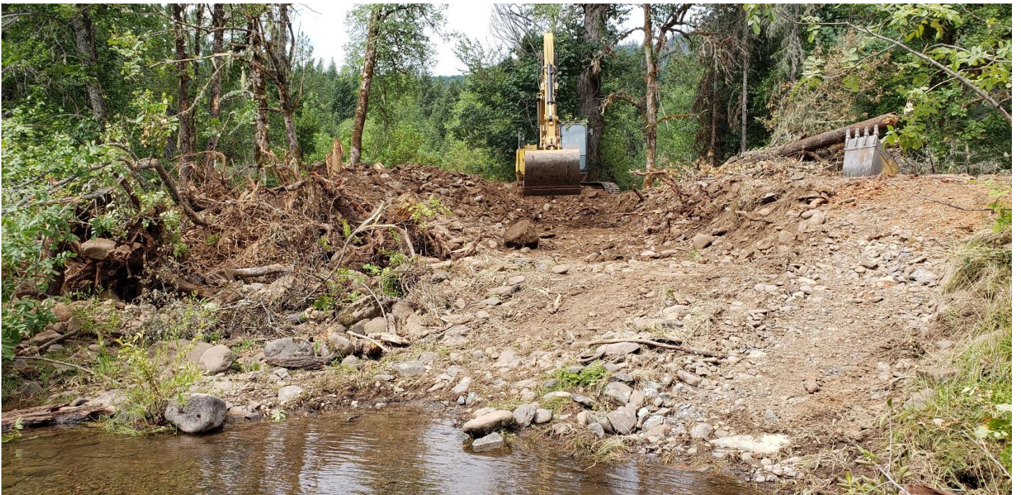
Excavating the artificial berm at inlet of side channel
